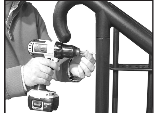
Step 9: Secure handrails using 1- #10 x 1 1/4" screw into each post at pre-marked locations.
