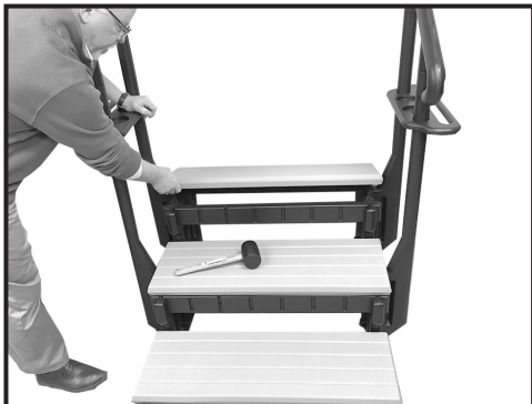
Step 10: Install the steps (finished edge out) by placing over the male lugs on the step sidewall and hitting downward with a rubber mallet.
