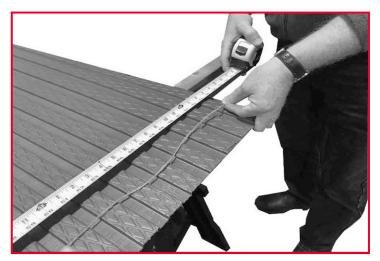
Measure the length of one of the spa panels and cut a piece of string to the exact length. The string will be used to layout the panels around the spa.
